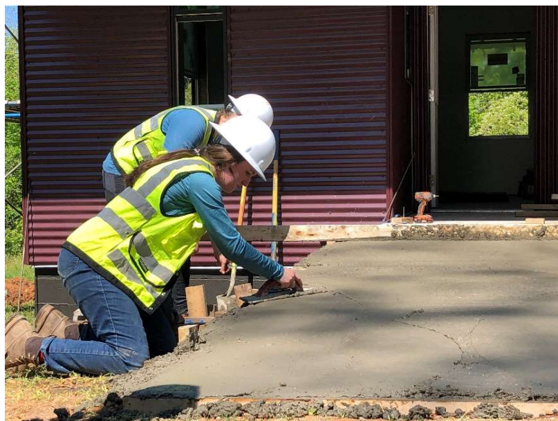
Smith constructing a ramp Ophelia's Home in Newbern, Alabama
